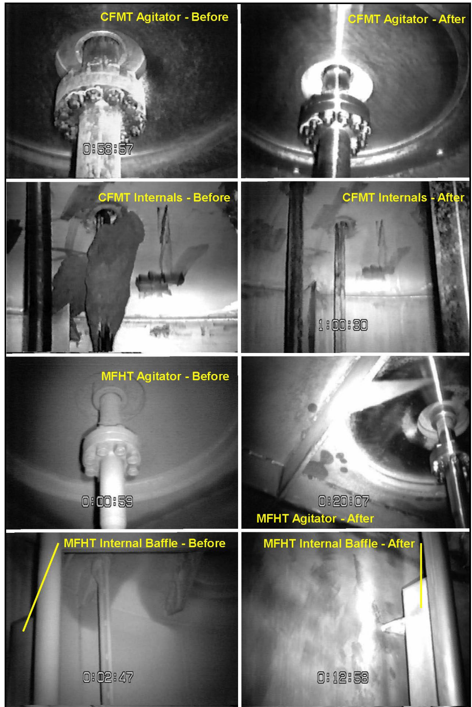
Figure 4-2. Before and After Flushing Images of the Two Vessels. (The shiny surfaces in the after images illustrate the effectiveness of the high-pressure washing in these WVDP photos taken with the underwater camera.) (from WVNSCO 2002c)
